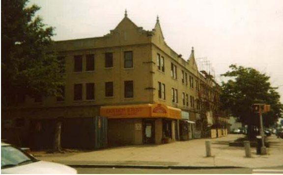
Weaver Building - Before
